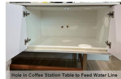
Hole in Coffee Station Table to Feed Water Line
